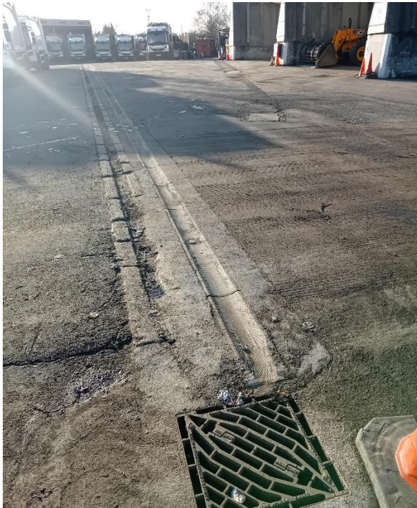
Figure 5. Reinstated drainage channels looking up the site
