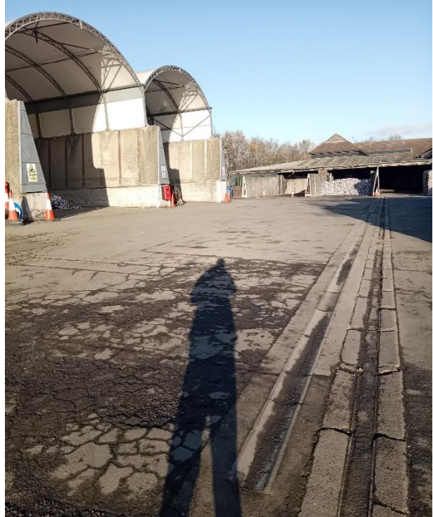
Figure 2. Reinstated drainage channels along length of the site
