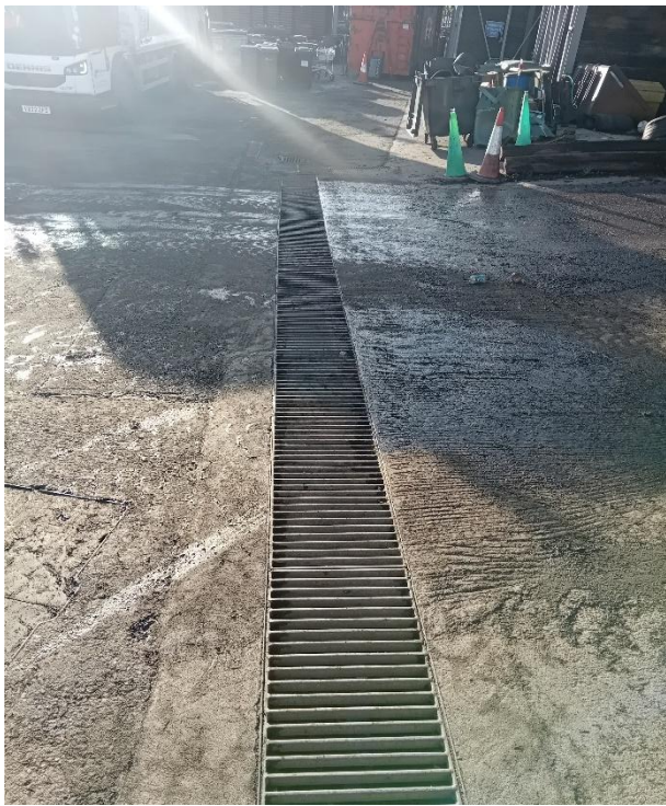
Figure 3. improved drainage channel adjacent to the street sweeping a electrical bay
