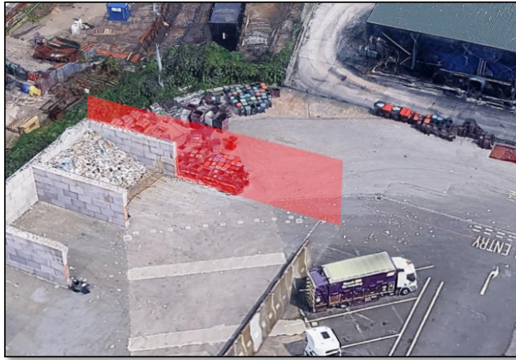
Figure 2 Firewall located at the end of the fibre bay storage area
