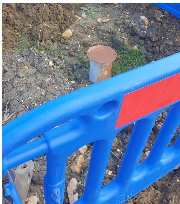
BH8540 - Pre condition
