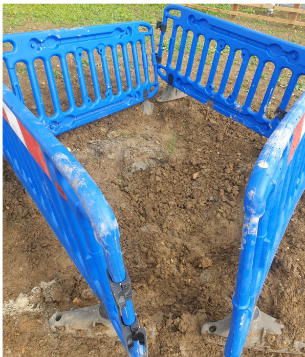
BH8540 - Post condition
