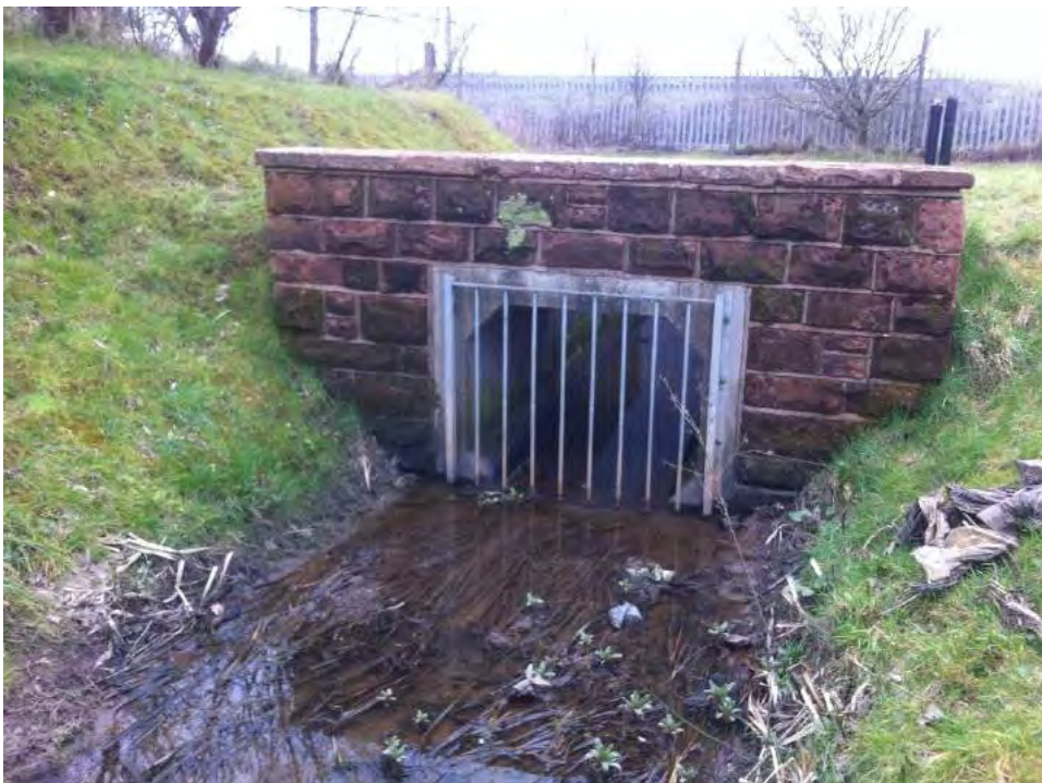
Figure 3-3 Trash screen on Cargo Beck to the north west of the Application Site
