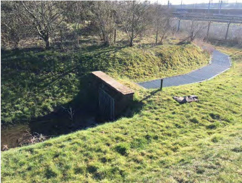
Figure 3-5 Concrete lined channel with metal grid roof to the north west of the Application Site
