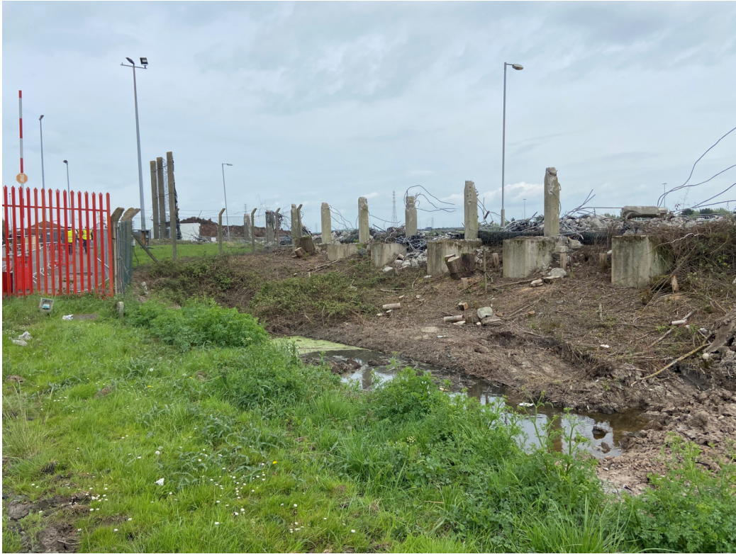
View NE from Redland Avenue.
