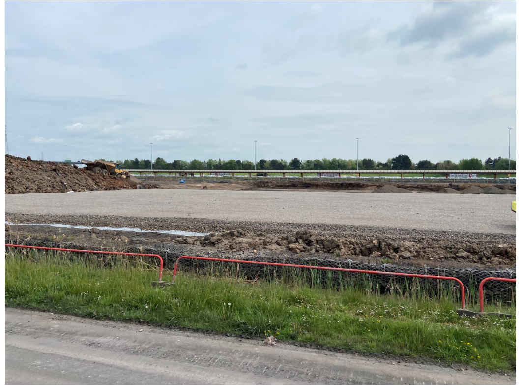
View S of pile mat under construction.
