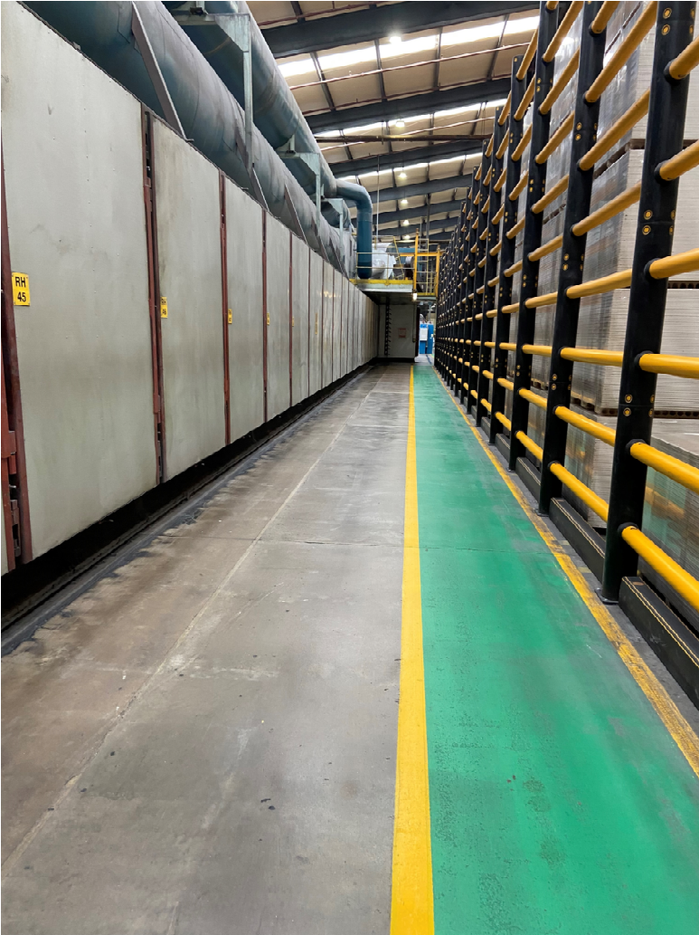
View along gas oven, hardstanding floor, impact barrier to right
