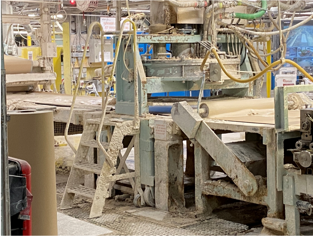
Plaster extrusion point
