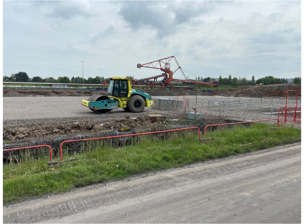
Pile mat under construction.
