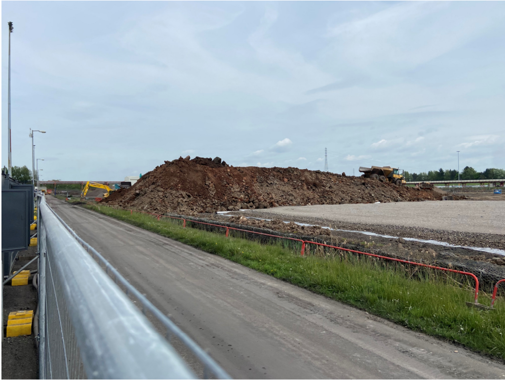
View E of stockpiled materials
