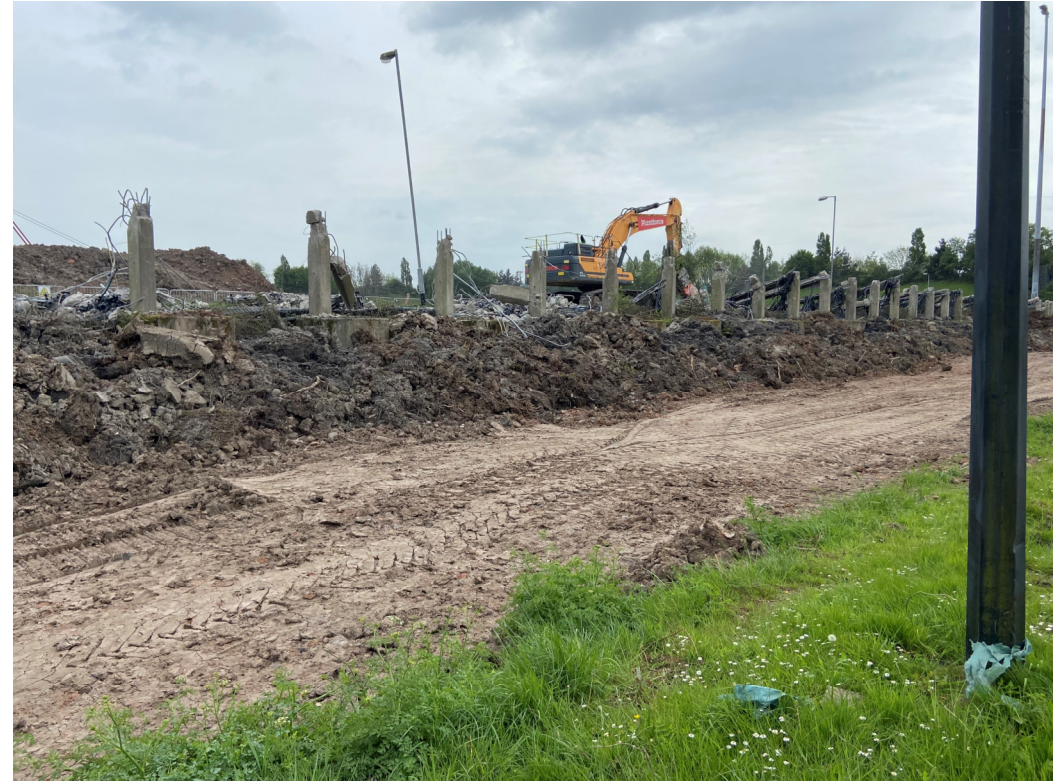
View SW from Redland Avenue.
