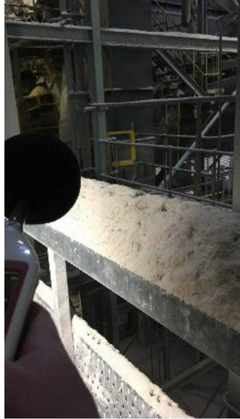
Conveyor near wall
