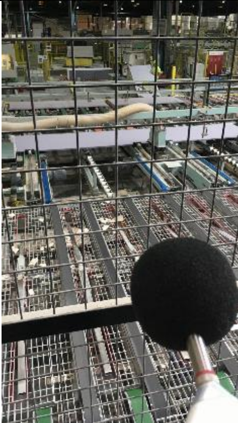
Bridge above cutter
