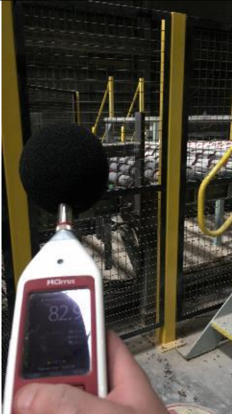
Conveyor from oven to cutter
