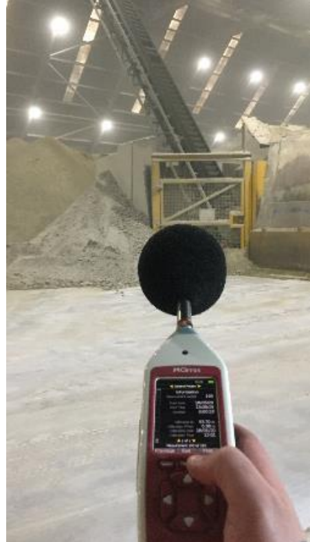
Conveyor centre of gypsum storage
