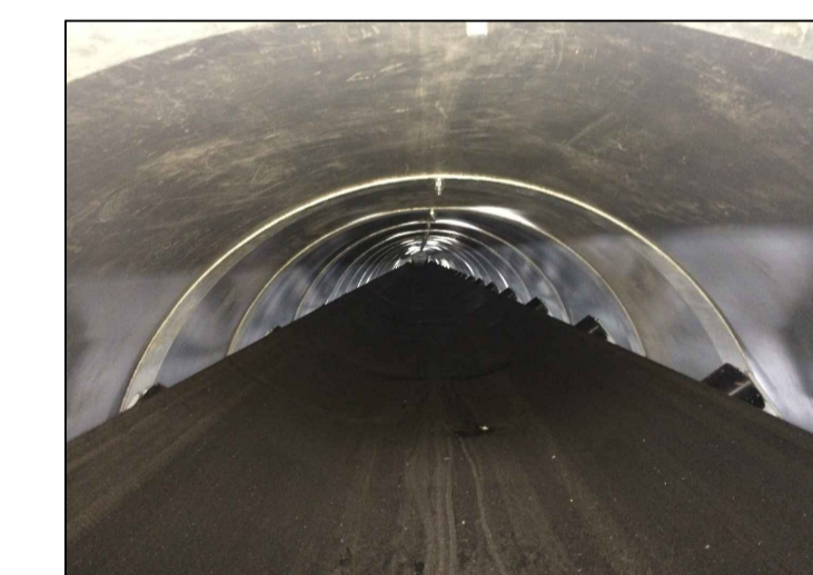
View Inside Of Covered Belts
