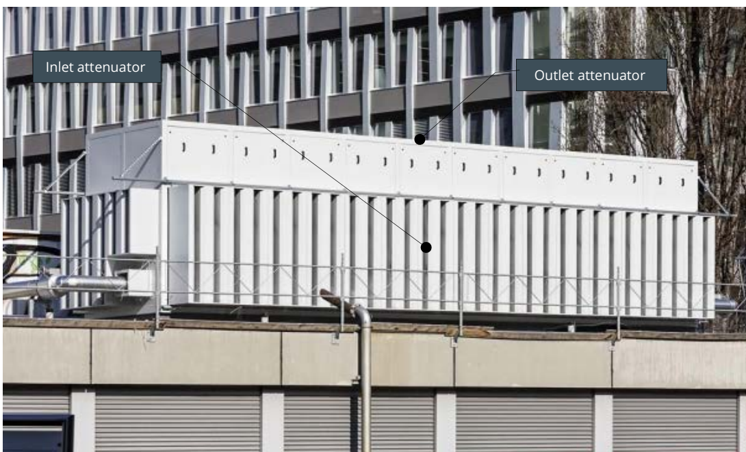
Figure 9: Example of acoustic attenuator AA303S
