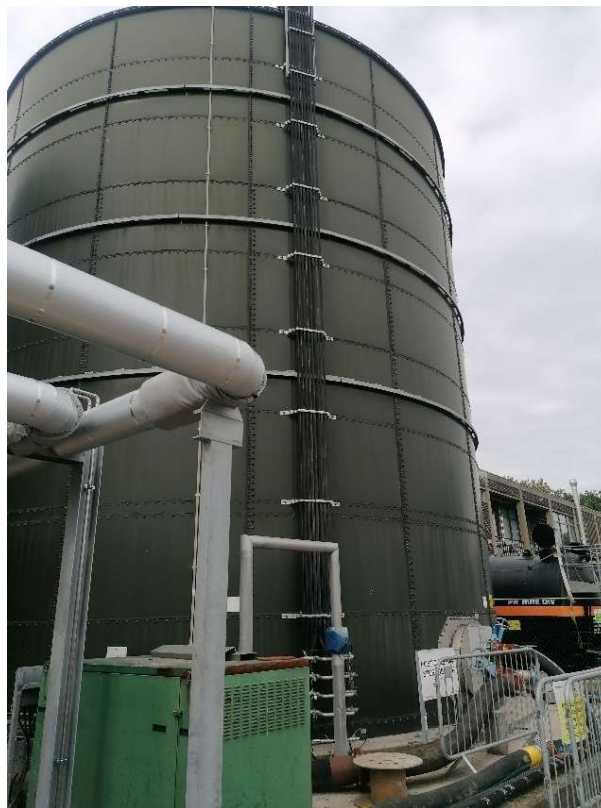
Figure 8.2.1 Post Digestion Tank
