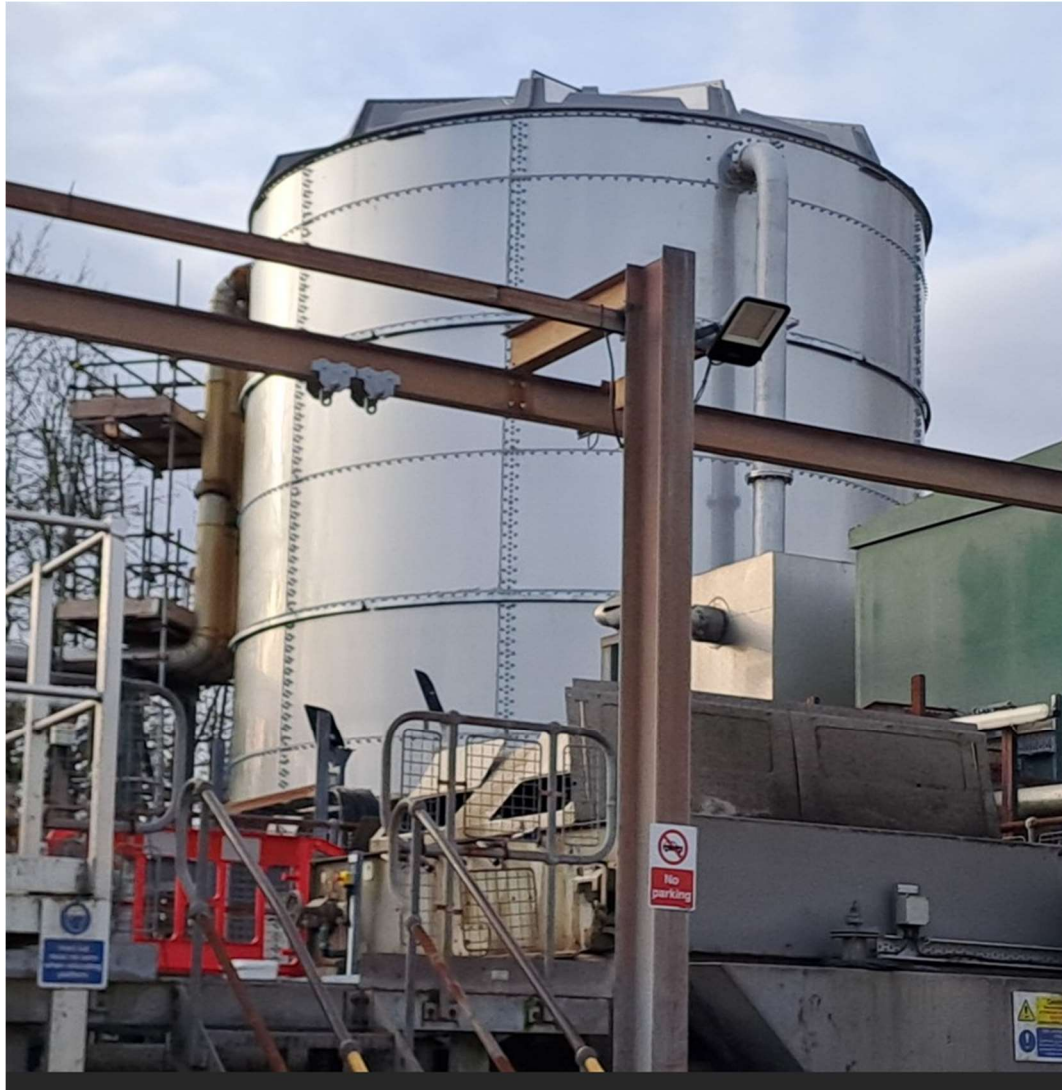
Figure 8.14: APD GBTs 1, 2 and 3 Feed Tank
