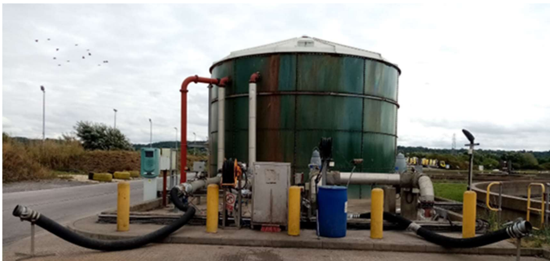
Figure 8.6: Imported Sludge Reception Tank Showing the Shallow Reinforced Concrete Bund, and External Pipework.
