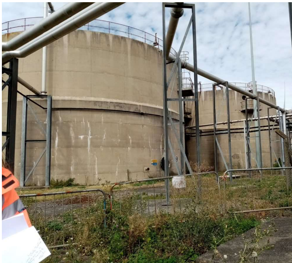
Figure 8.19: Mesophilic Anaerobic Digester P6
