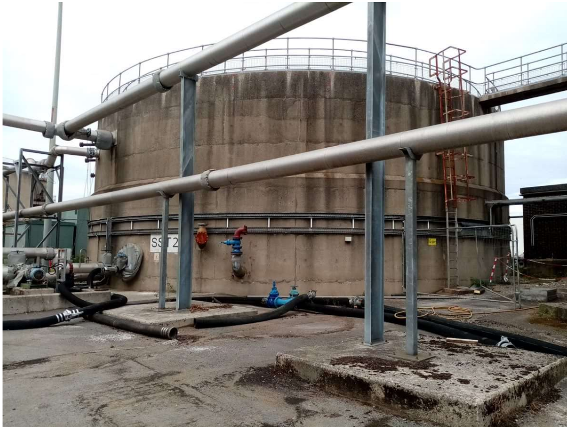
Figure 8.21: Secondary Sludge Storage Tank (SST2)
