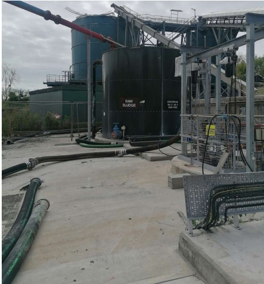
Figure 8.25: Centrifuge No.5-No.6 Raw Feed Tank
