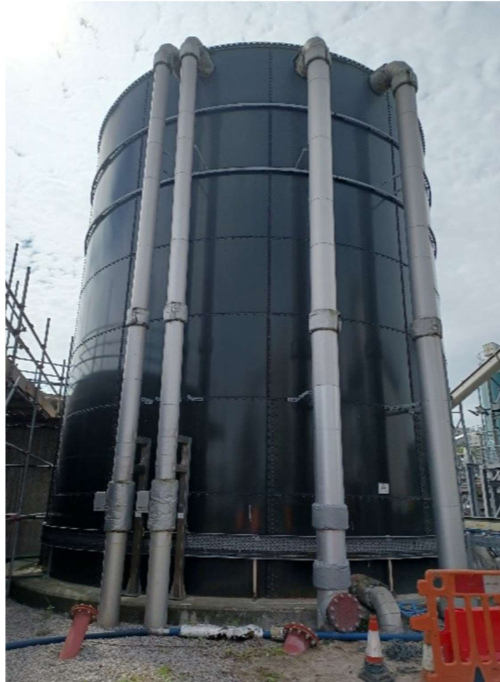
Figure 8.23: Centrifuge Feed Sludge Tank
