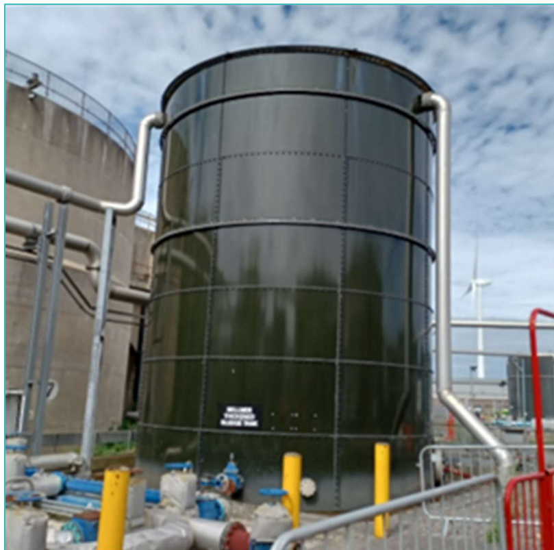
Figure 8.12: Bellmer Thickened Sludge Tank
