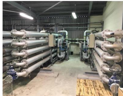
Figure 6: Heat exchangers
