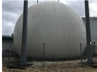
Figure 7: Double membrane gas bag
