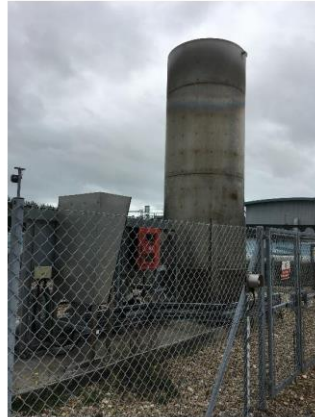
Figure 9: Flare stack area
