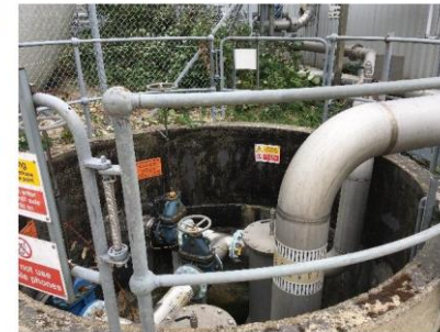
Figure 8: Gas condensate pit
