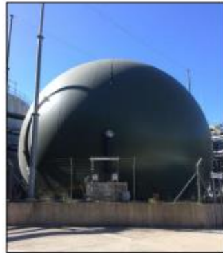
Figure 18: Double membrane gas bag.
