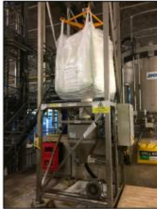
Figure 11: Polyelectrolyte dispenser 3.
