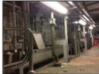
Figure 2: Inlet screening.
