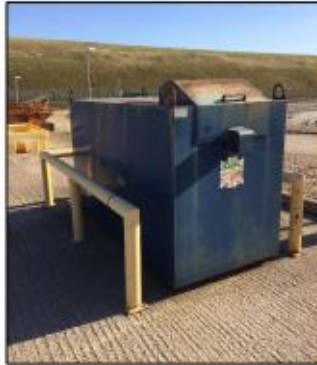
Figure 25: Permanent diesel tank.
