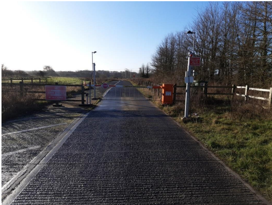
B3073 entrance barrier
