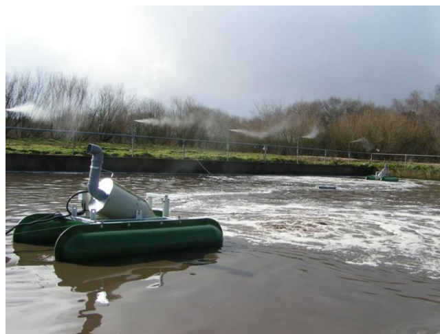
Plate 4 Photographic Plate of Lagoon Aeration Pumps
