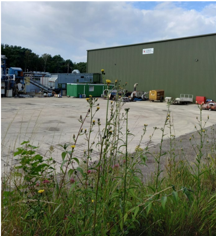
Image EDP A1.1: Hardstanding and main structure within the EfW CHP Facility Site
