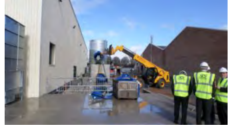
Guests at the opening of the plant in 2014
