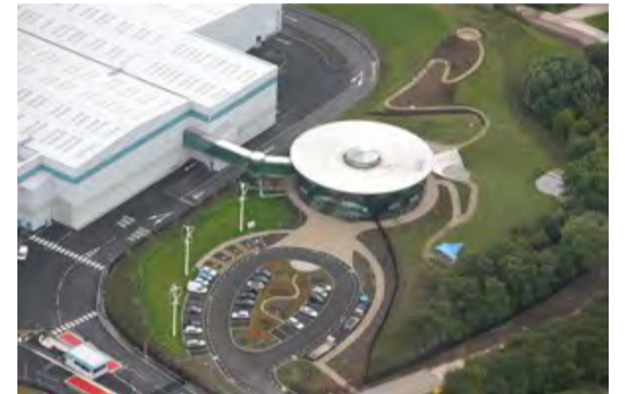
Global Renewables Farington MBT facility is now jointly owned by Lancashire and Blackpool councils
