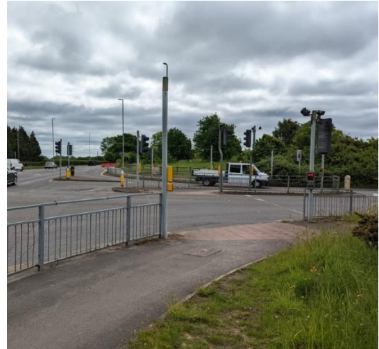
Photograph 7: Signalised pedestrian crossing (S)
