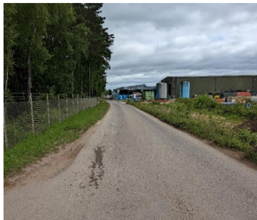
Photograph 3: Service Road along northern boundary of the EfW CHP Facility site
