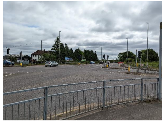
Photograph 7: Signalised junction from SW corner
