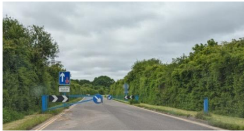
Photograph 1: Traffic Calming on Arena Way
