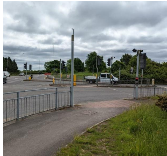
Photograph 9: Signalised pedestrian crossing (S)
