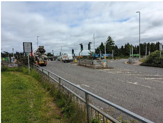
Photograph 6: Signalised junction from Arena Way
