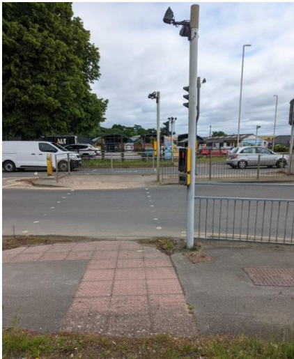
Photograph 8: Signalised pedestrian crossing (W)
