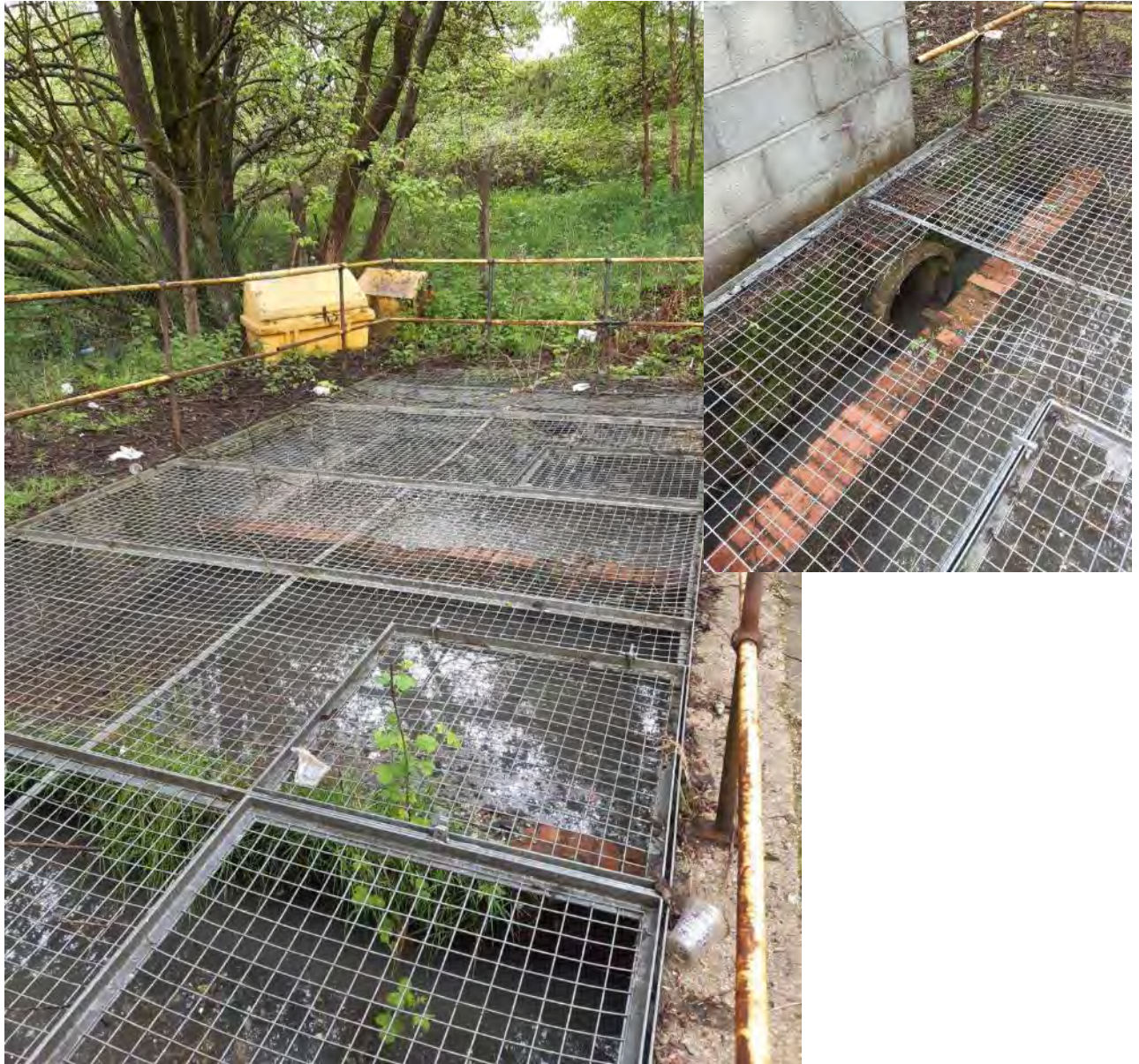
Plate 5, Interceptor with closeup of outfall pipe (inset)
