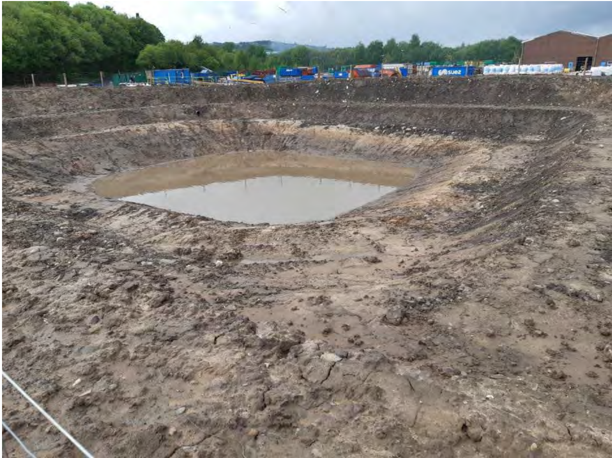
Plate 11, New fire water pond under construction in east of the site
