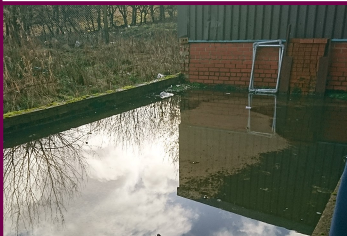
Photo 23: Brick bund adjoining north of building
