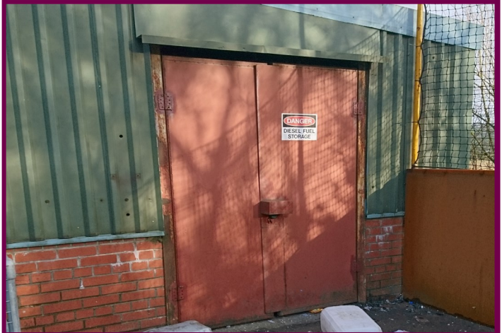
Photo 22: Building containing diesel tank
