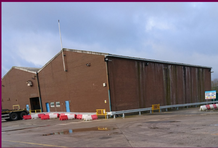
Photo 11: Warehouse in centre of site
