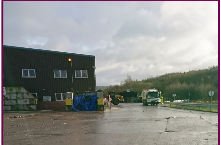
Photo 10: Warehouse in north east of site
