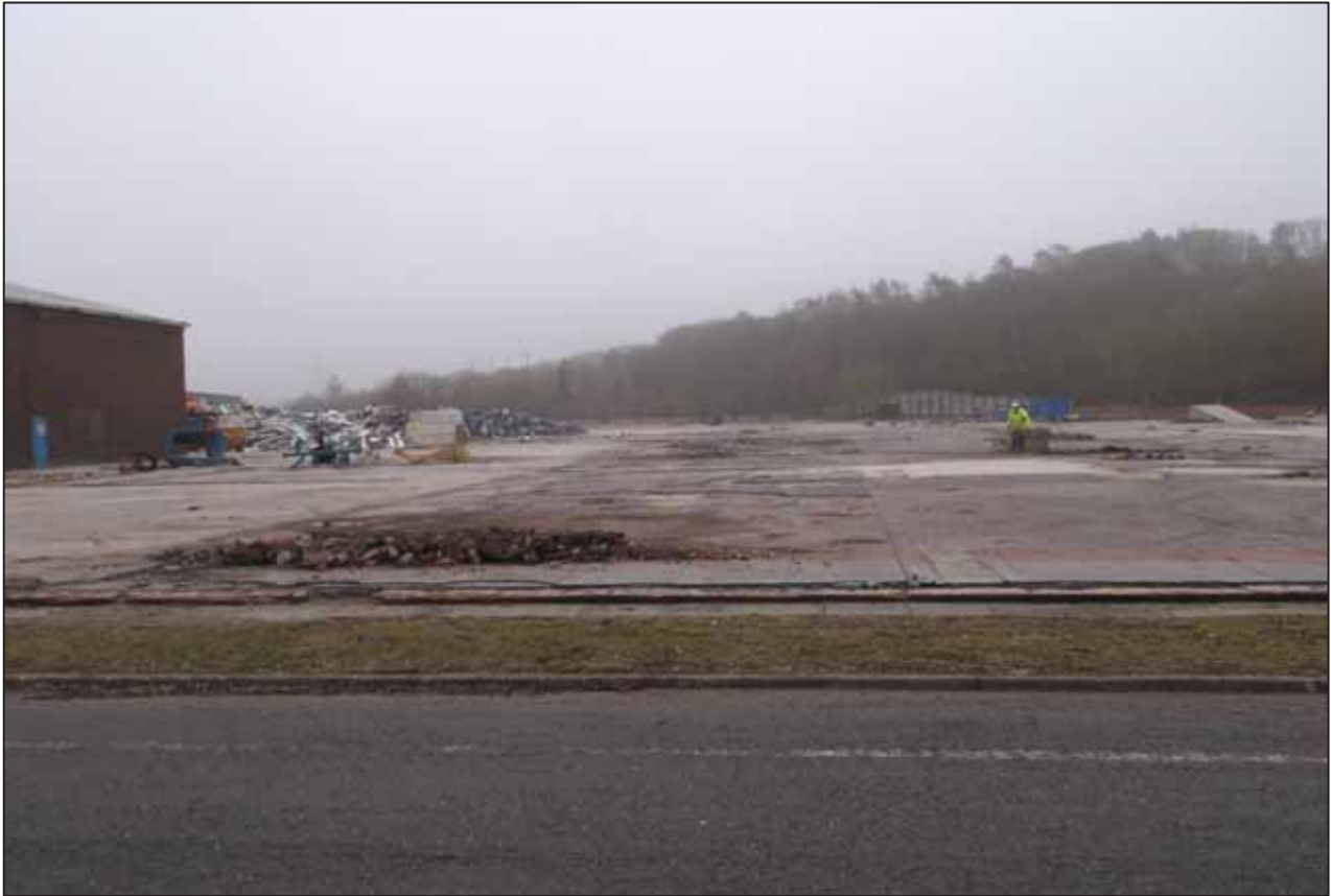
Photograph 13: Looking east across the northern area of the proposed WTF facility
