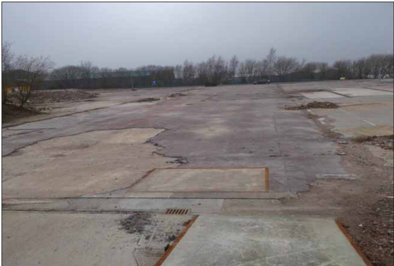
Photograph 10: Looking west across the southern area of the proposed WTF facility
