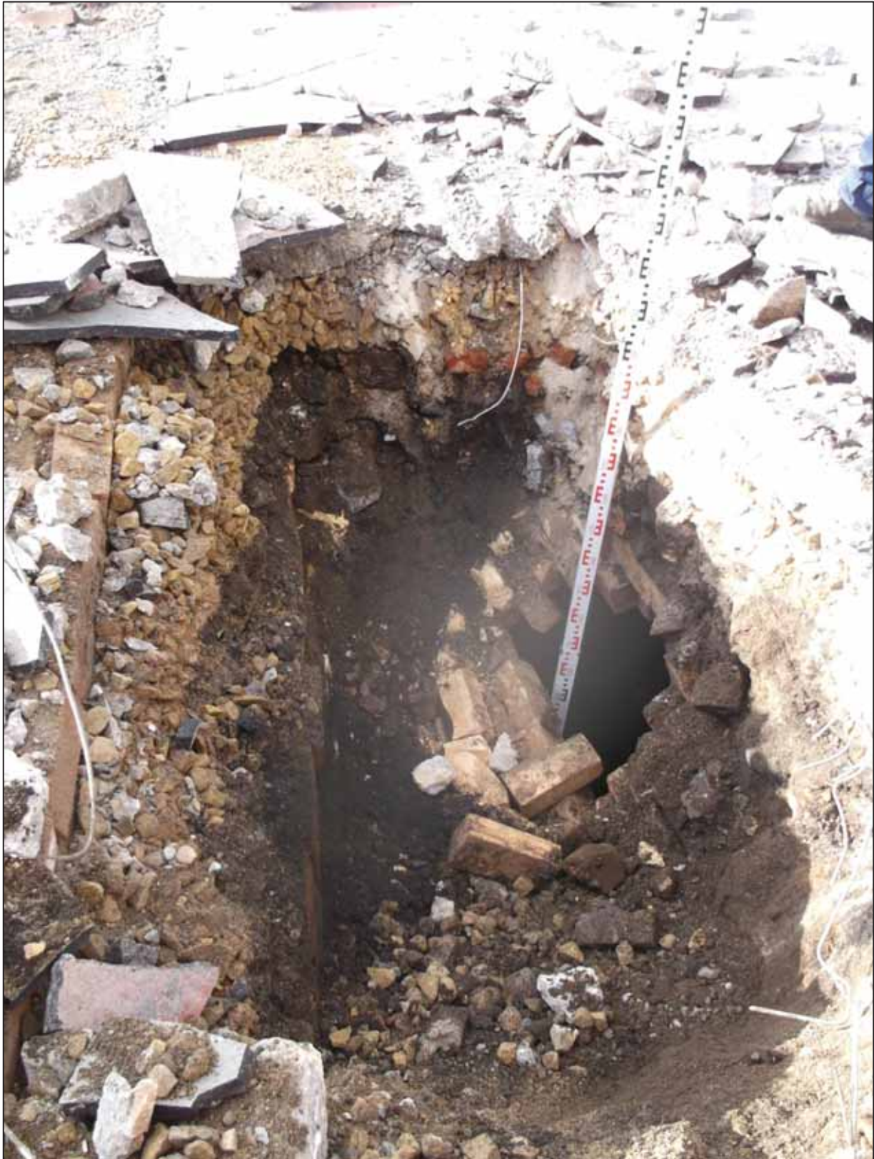
Photograph 2: Trial Pit TP3
