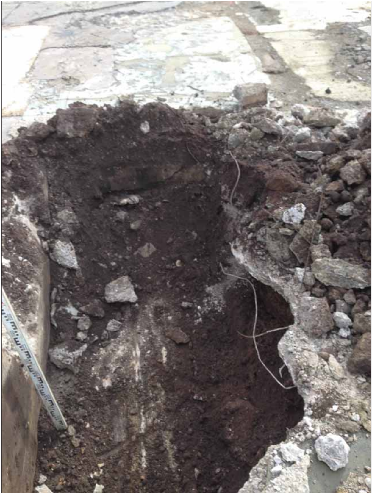
Photograph 6: Trial Pit TP12
