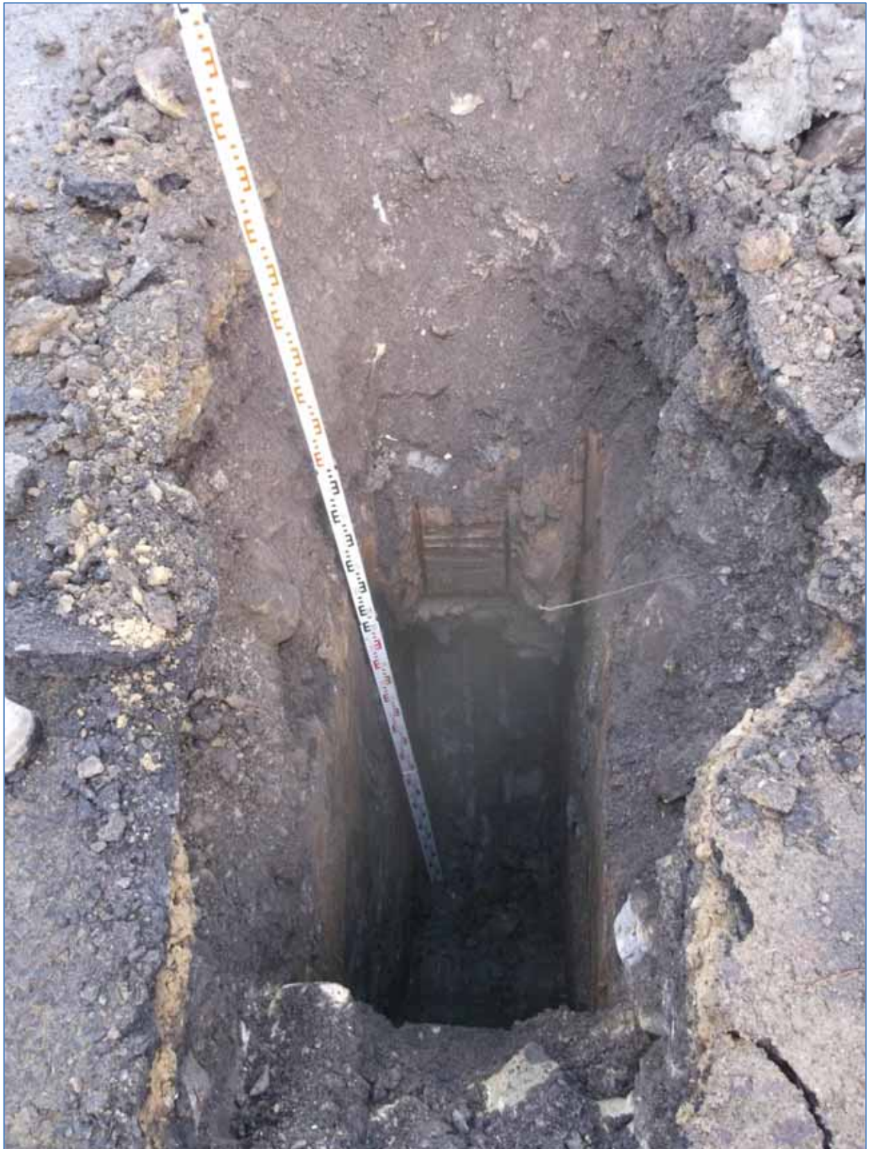
Photograph 1: Trial Pit TP2
