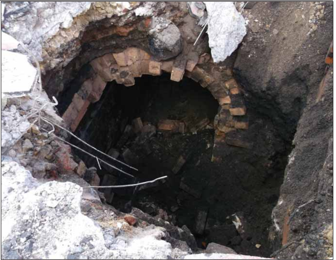
Photograph 3: Trial Pit TP3
