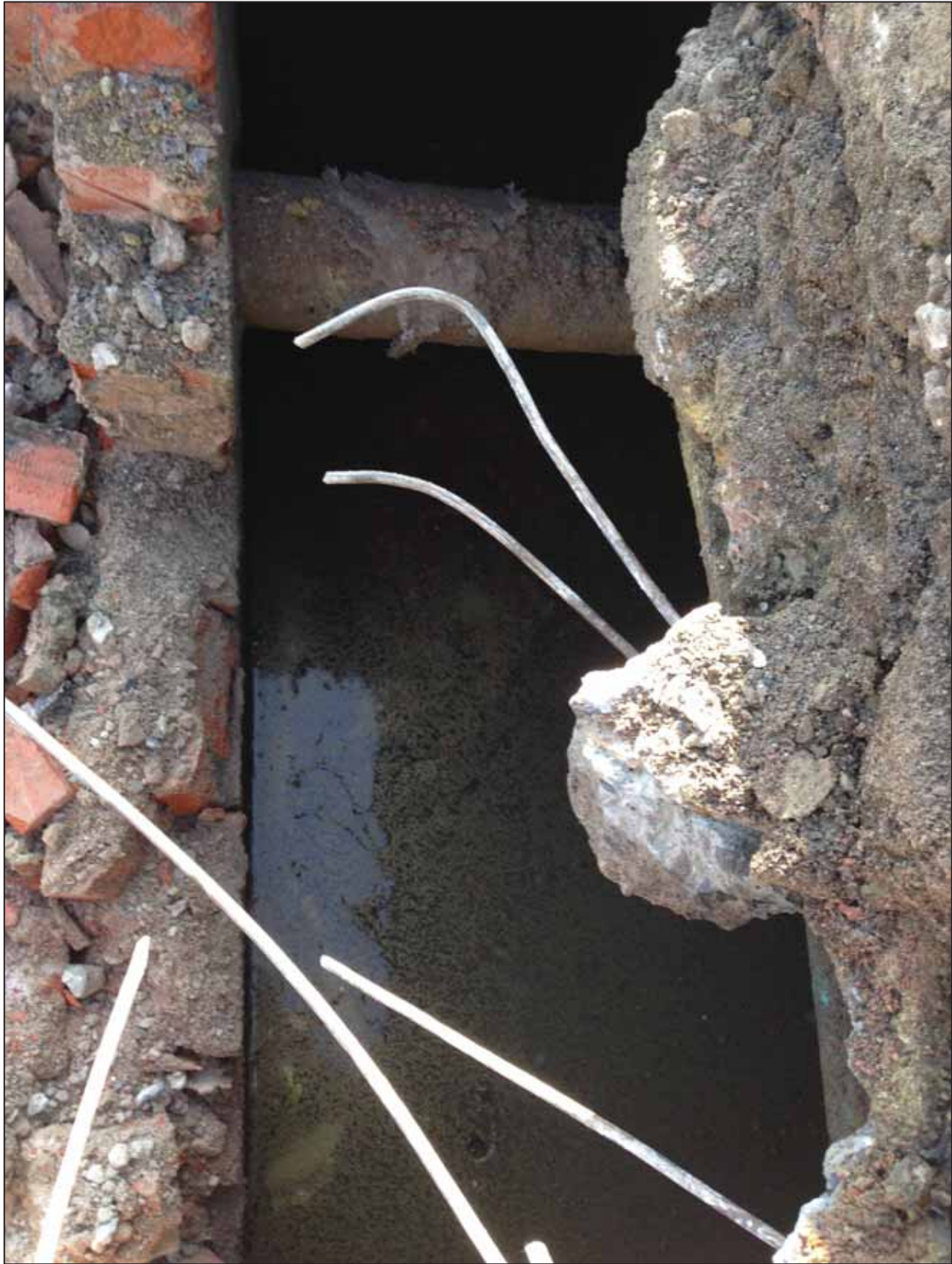
Photograph 7: Trial Pit TP16 (suspected old water tank)
