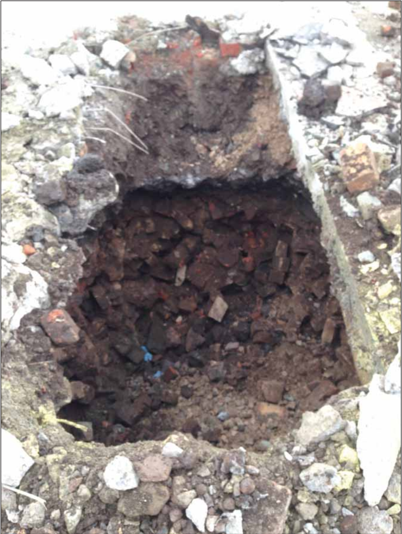
Photograph 4 Trial Pit TP6
