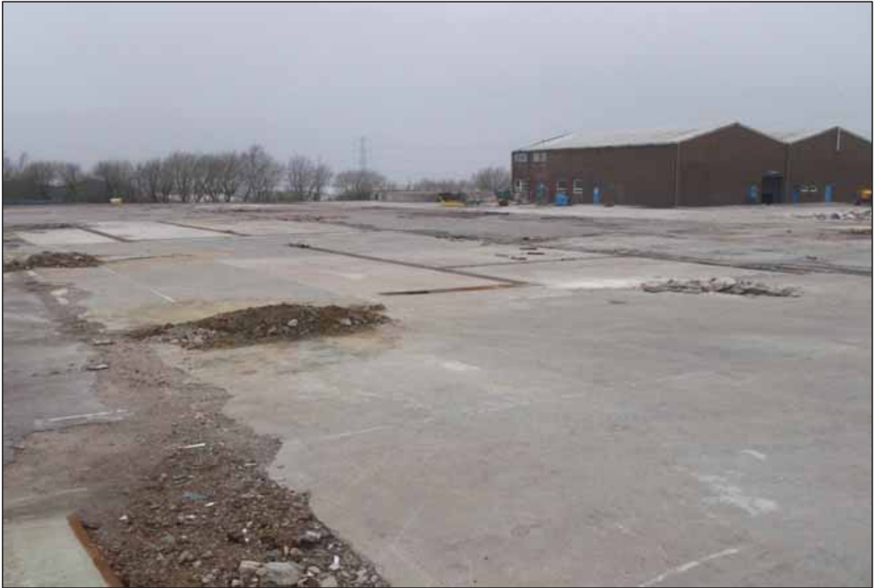
Photograph 11: Looking north east across the area of the proposed WTF facility
