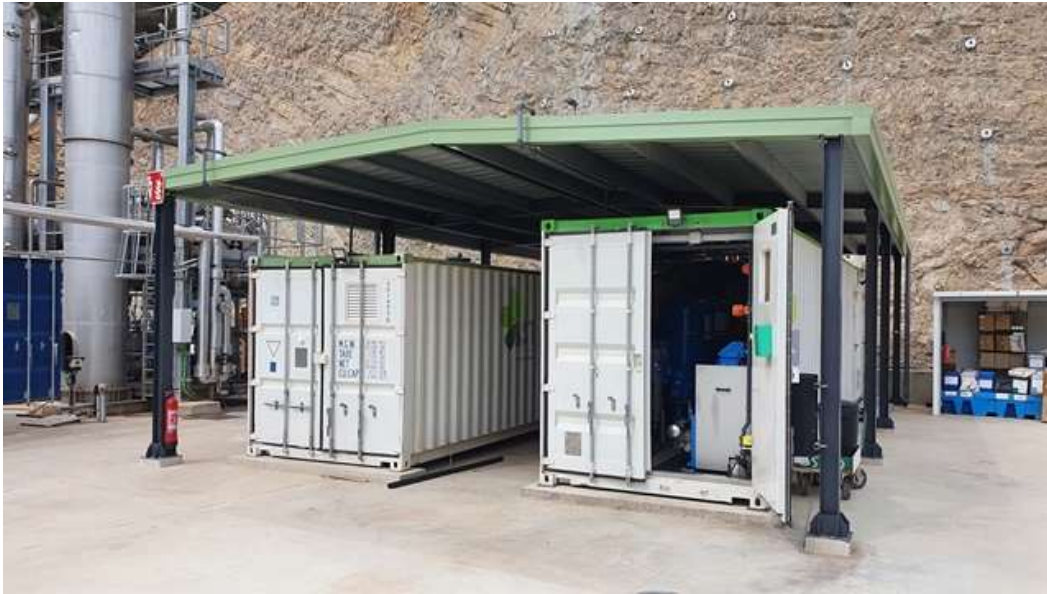
Figure 12. RO Leachate System treatment in three stages, flow rate of 250 m 3 /d, and OR System for concentrate reduction followed by evaporation, Ibiza, Spain.
