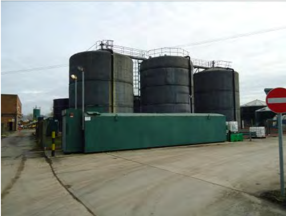
Photo 3 Existing sludge storage tanks
