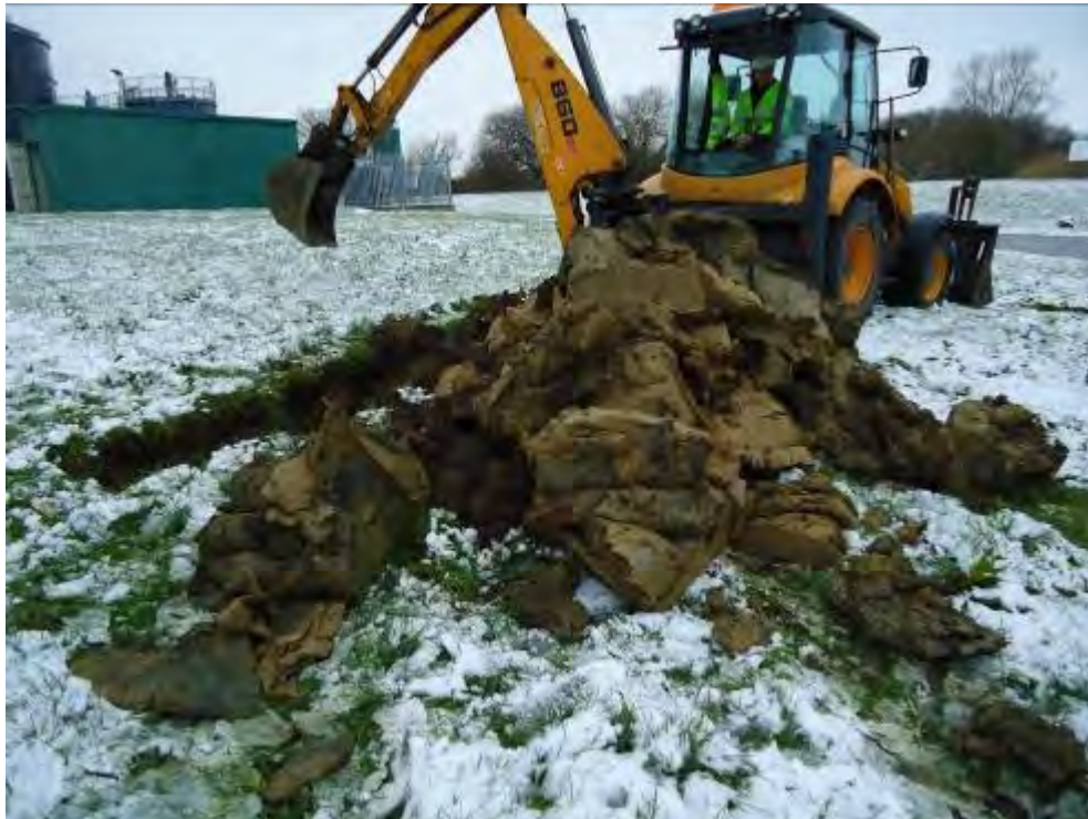
Photo 21 Spoil from TP5
