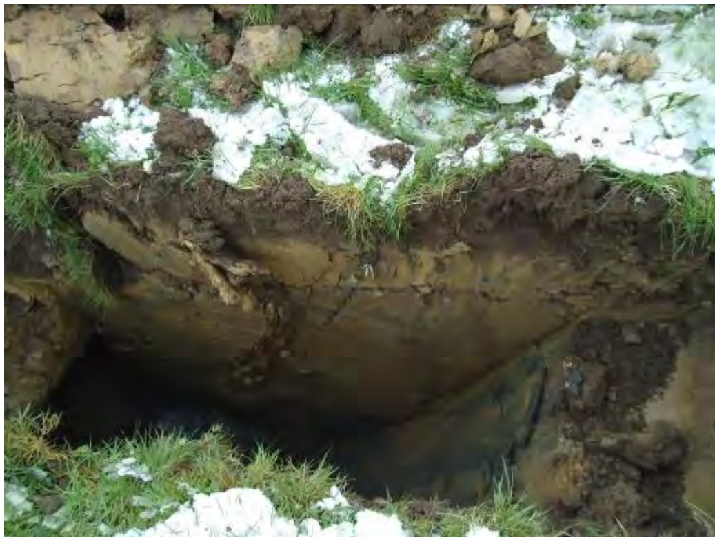
Photo 18 Side of TP5
