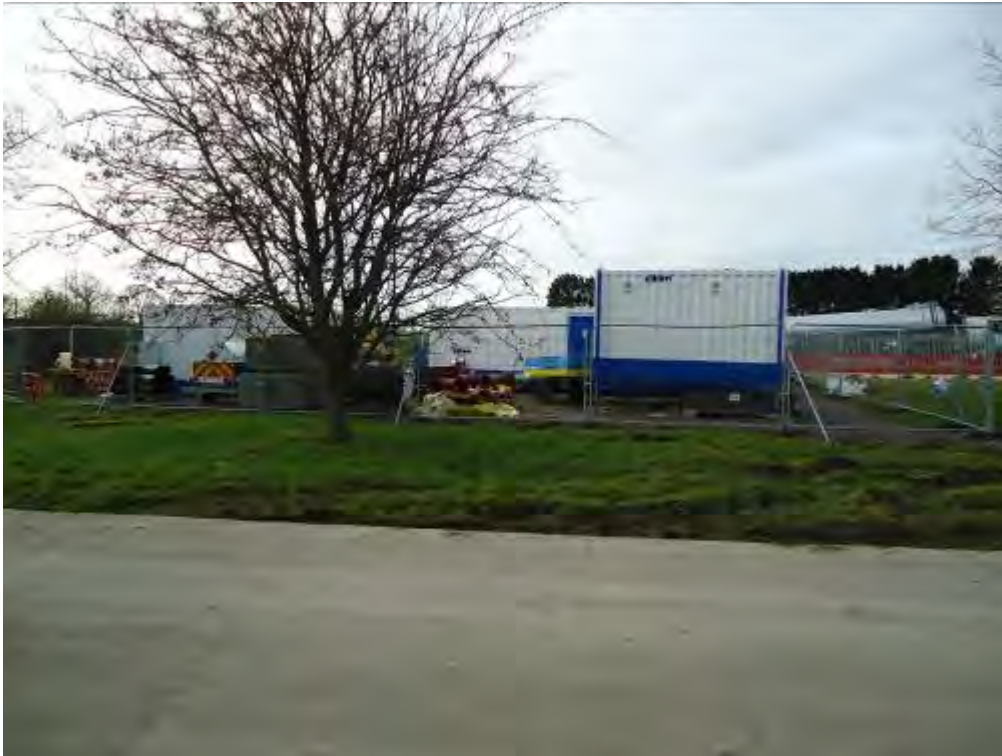
Photo 5 Location of BH2 and Balfour Beatty contractors on site
