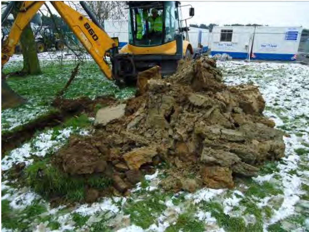
Photo 26 Spoil from TP6
