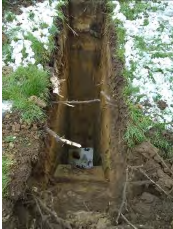
Photo 25 Front end of TP6
