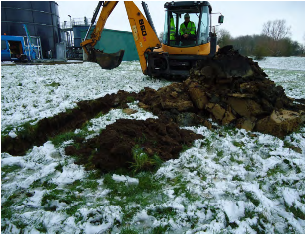
Photo 16 Spoil from TP4
