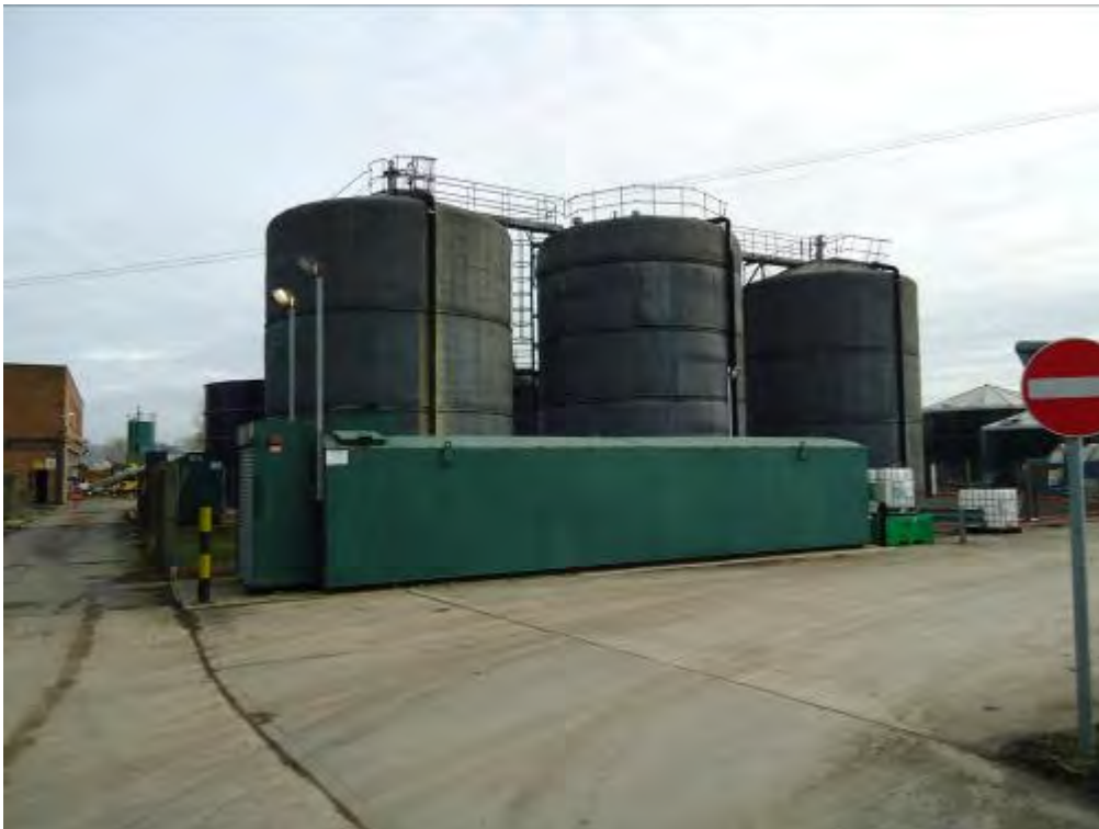
Photo 3 Existing sludge storage tanks
