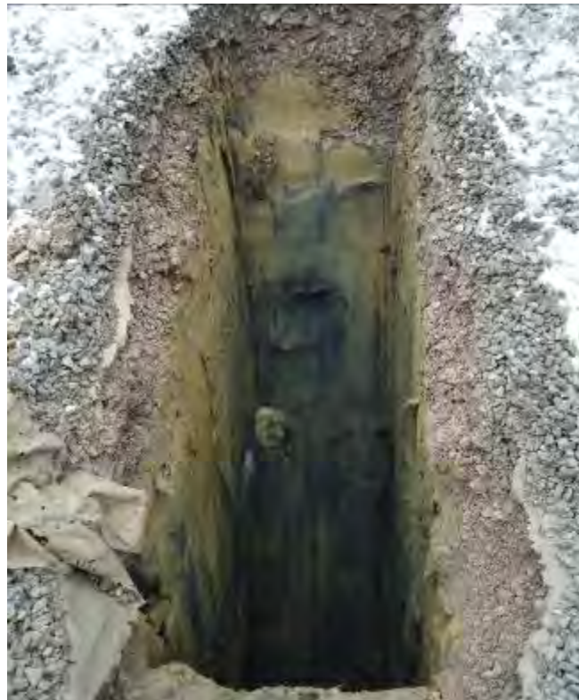
Photo 10 Front end of TP3
