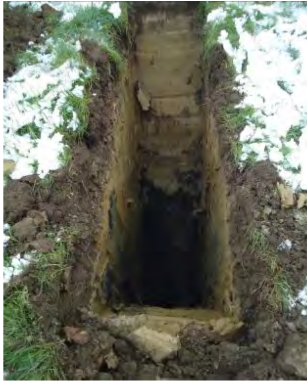
Photo 15 Front end of TP4
