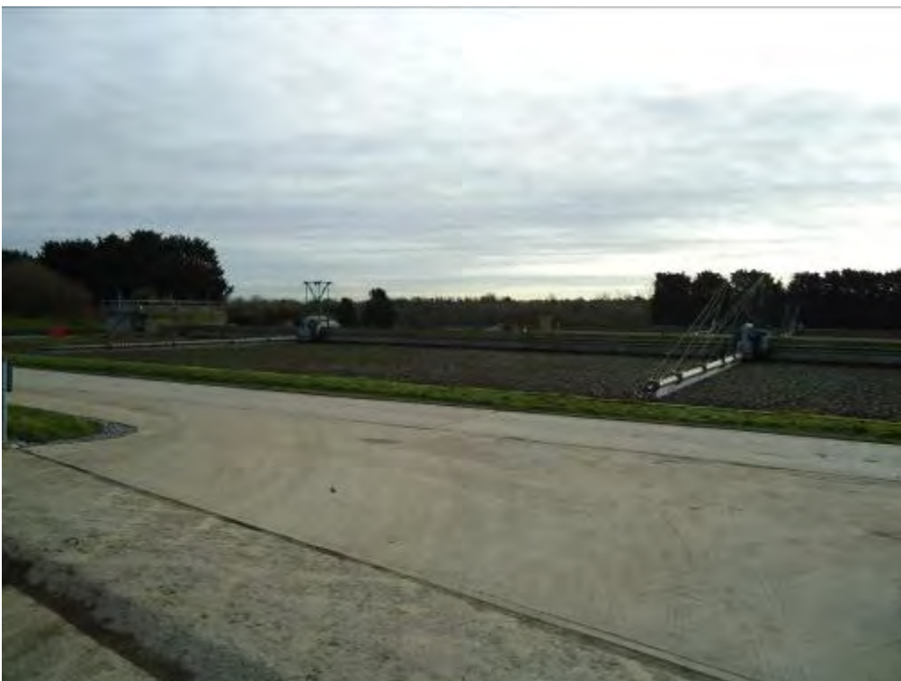
Photo 4 Filter beds located to the south east of site
