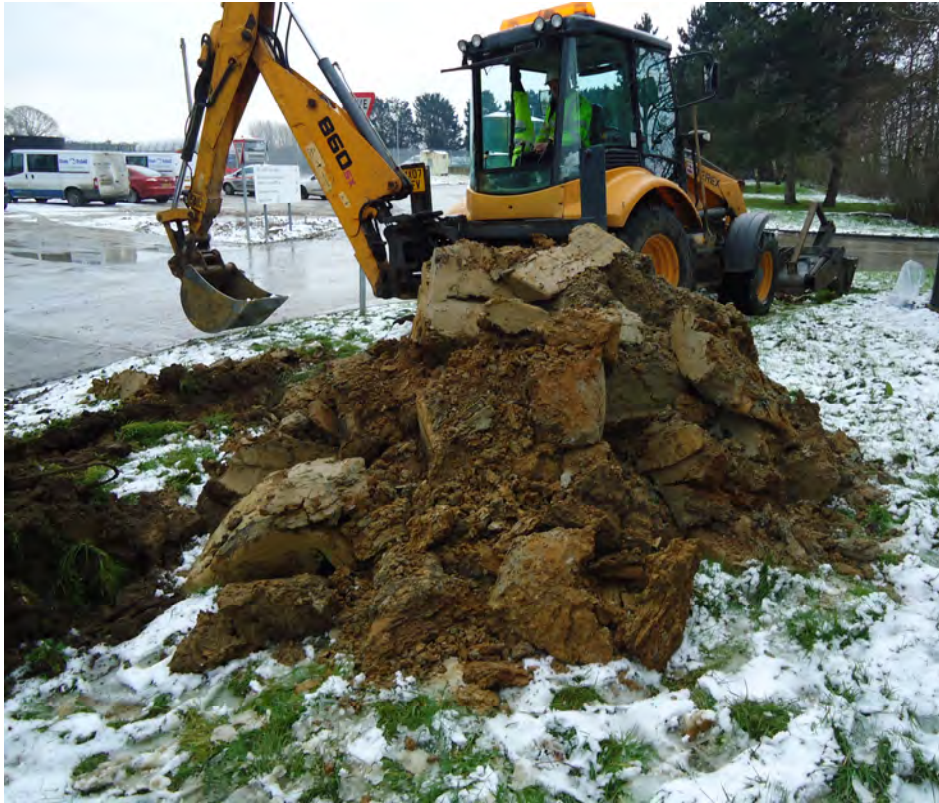
Photo 5 Spoil from TP2
