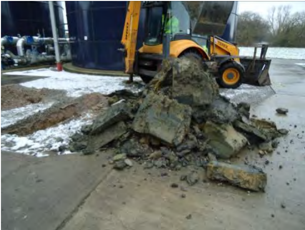
Photo 11 Spoil from TP3
