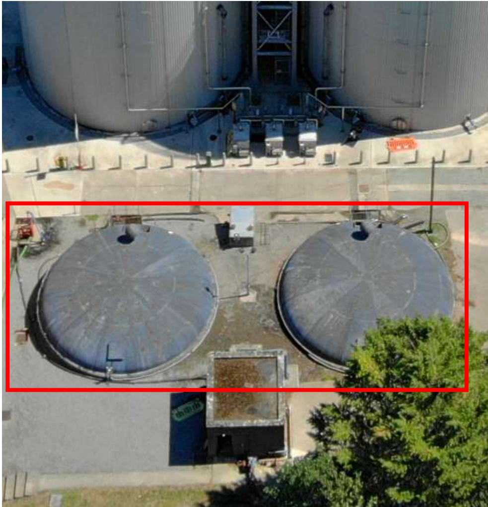
Figure 8.15 Liquor Balancing Tanks
