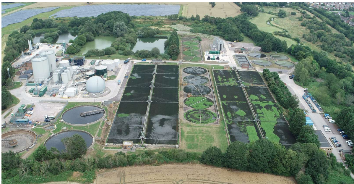
Figure 8.1 Trowbridge WRC and STC
