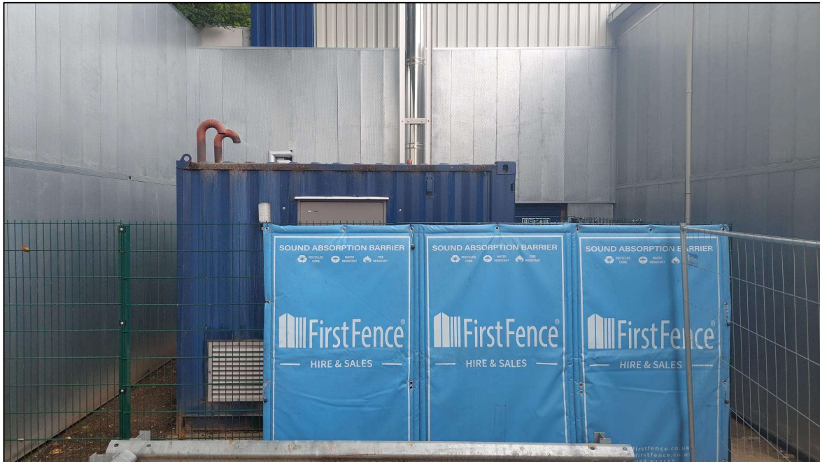
Figure 1 - Noise Mitigation Measures around Boiler Plant
