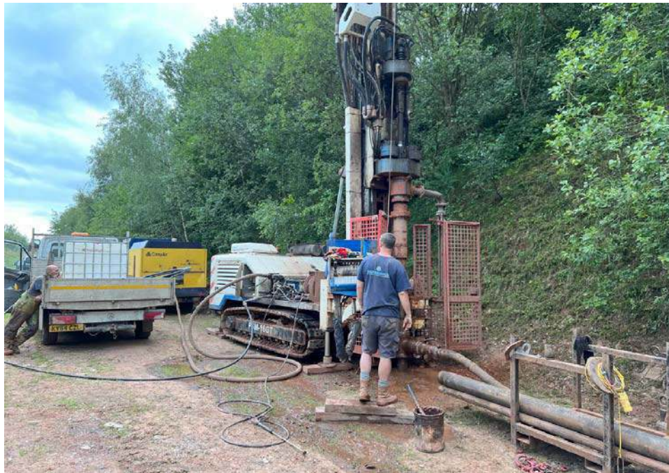
Plate 1: View of borehole ESID4 being drilled using PSM 166T drilling rig.
