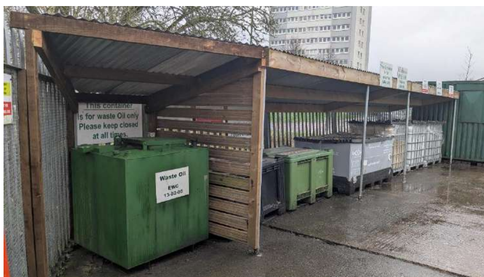
Plate 7: Double Skinned Waste Oil Storage Tank
