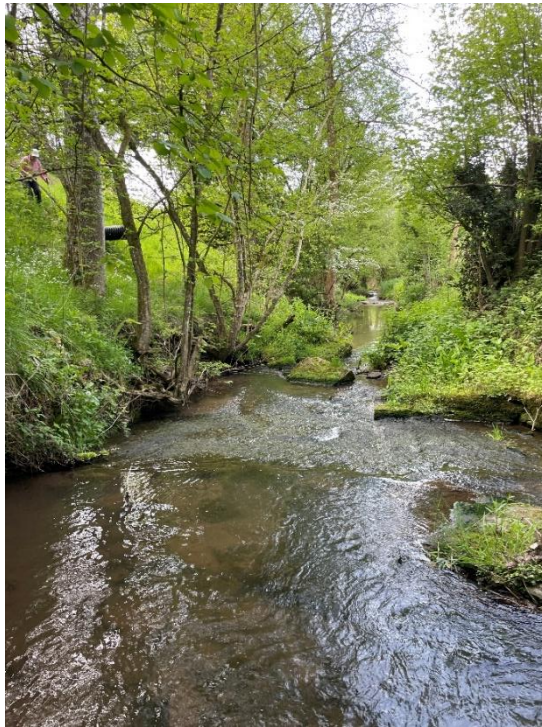
Figure 3. Steep gradient of the riverbed, approximately 30 m downstream of the failed weir.
