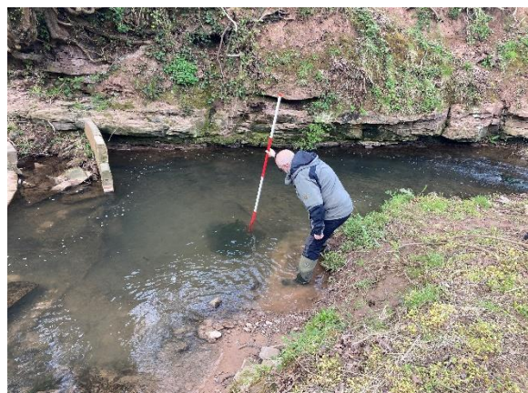
Figure 7 - Section of eroding cliff on the western bank and defunct weir.
