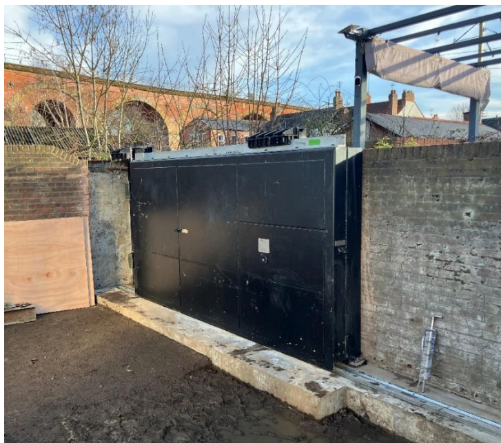
Figure 1. New sliding Gate 17 Installed
