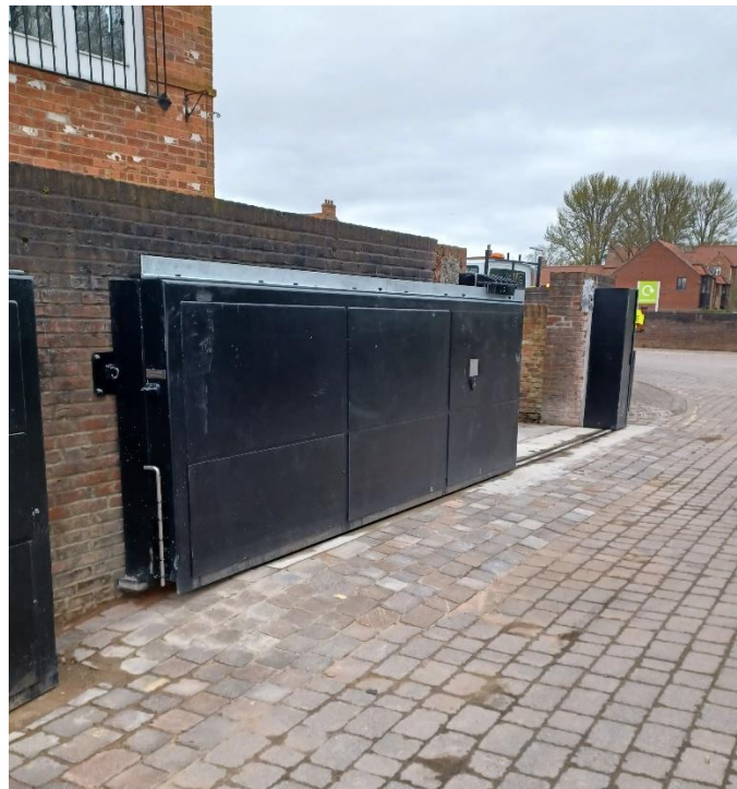
Figure 2. New sliding Gate 27 Installed and Tested
