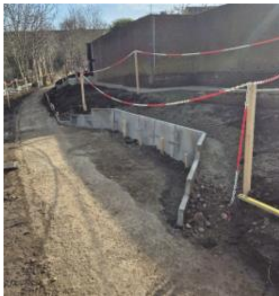
Figure 2. New passing places installed on True Lovers Walk – tarmac to be laid.
