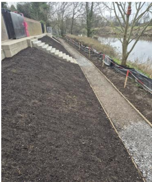
Figure 1. Reinstatement of embankments and footpath continues.
