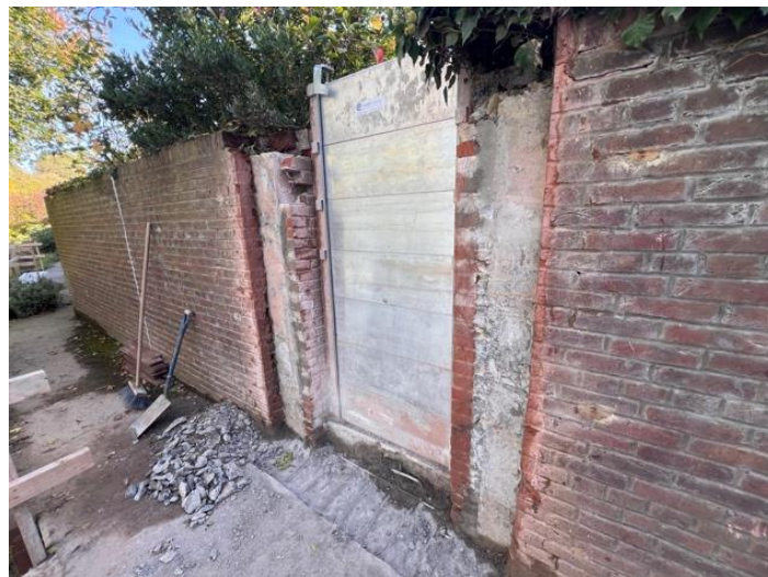
Figure 4. Gate 13 Temporary Flood Protection following removal of Flood Gate.
