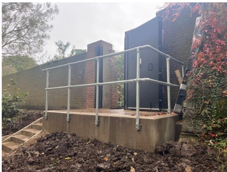
Figure 2. Gate 3 Access Steps and Handrails.
