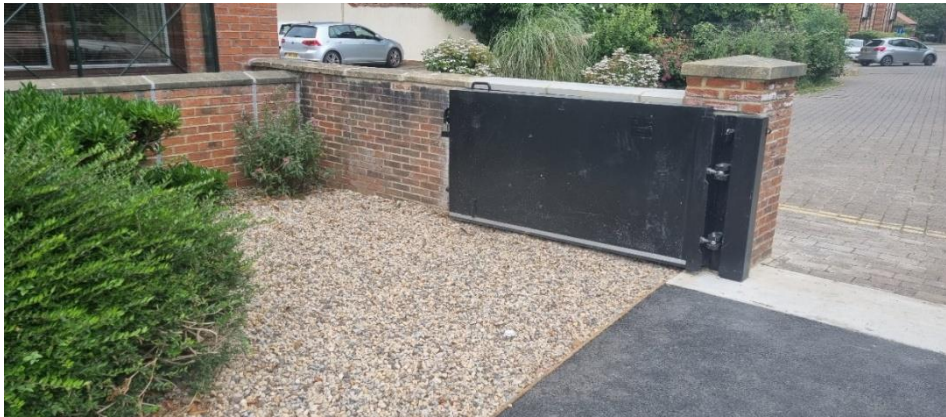
Figure 1. Gate 31 Installed and Tested
