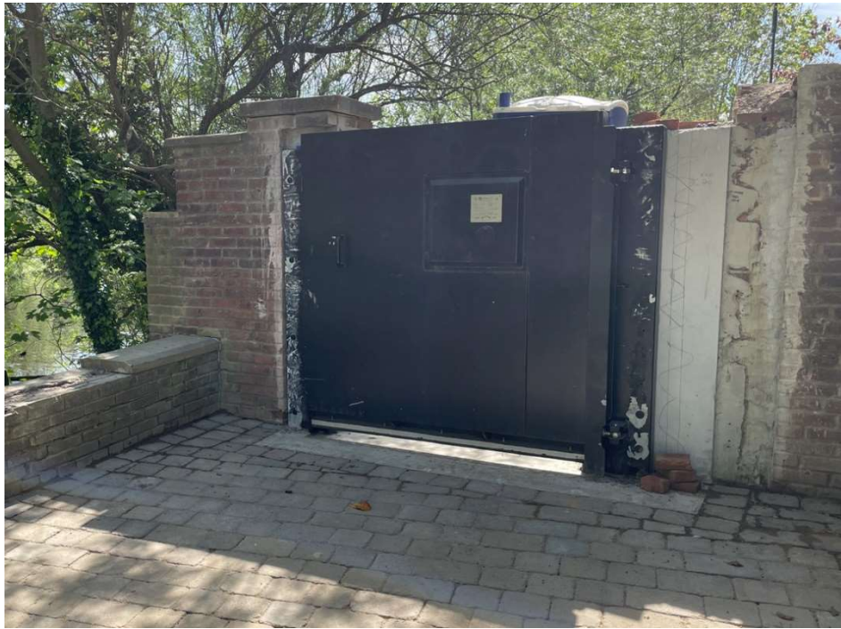
Figure 1. Gate 30 installed and awaiting brickwork cladding replacement.
