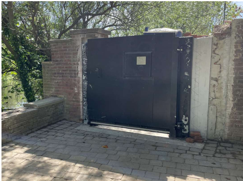
Figure 1. Gate 30 installed and awaiting brickwork cladding replacement.
