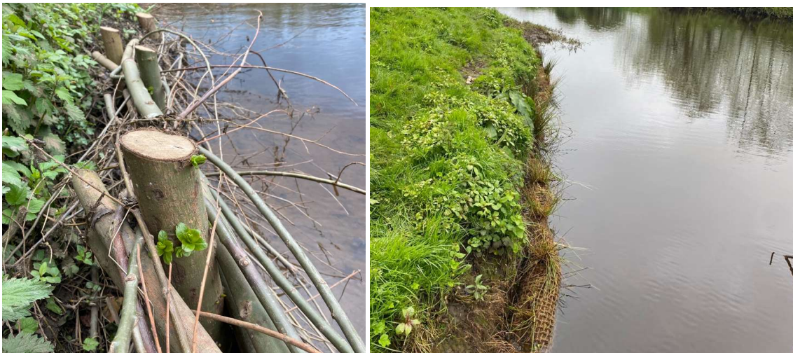
Figure 8&9. Environmental Enhancements - installation of willow spiling, enhancement of reed beds
