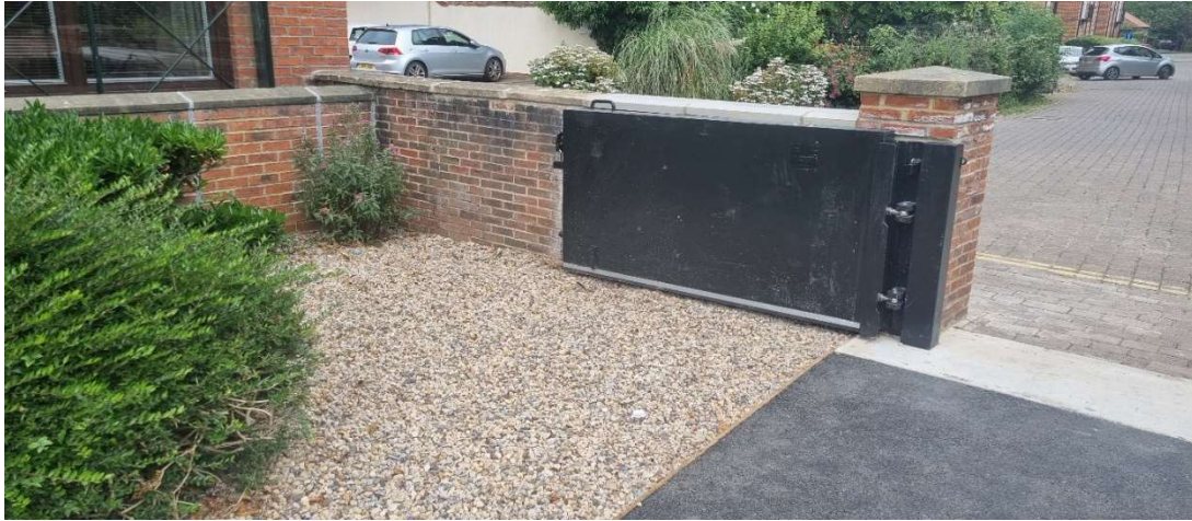
Figure 3. Gate 31 Installed and reinstatement completed.
