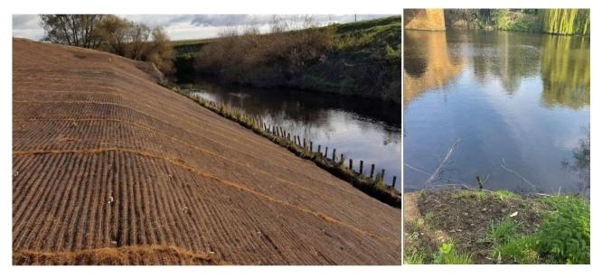
Location 3 is upstream of the road bridge. This area has had previous works installed which have now failed (see pictures right of the stakes). Replacement of the coir roll would be recommended coupled with some willow spiling to further reinforce the toe of the bank. The willow spiling will grow into the bank, strengthening the bank. The total length of this section is 15m.
