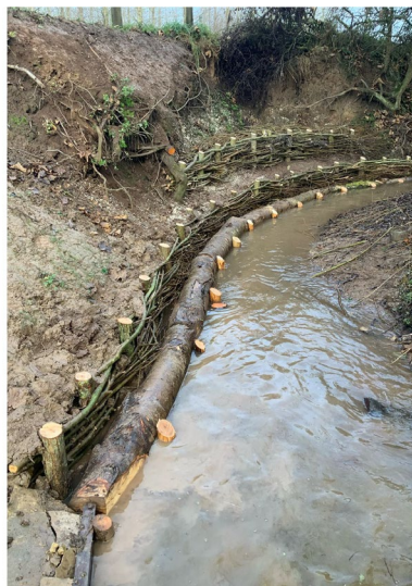
Figure 3. Example willow spiling completed by the Tees Rivers Trust
