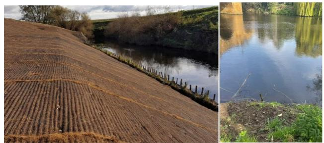
natural geotextile (coir type material) or bank reinforcement mesh to create a more purpose-built area for this activity. The lower edge of the bank could be armoured further either with a coir roll or using a timber edge (tree trunk or similar). The reinforced area of bank can then be seeded with a mixture of native and locally sourced plant species, creating valuable habitat.
