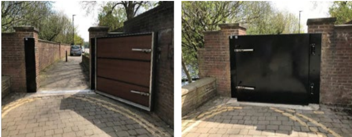
Figure 3 – Existing flood gate 30 showing the wood effect cladding which won't be on the new flood gates.
