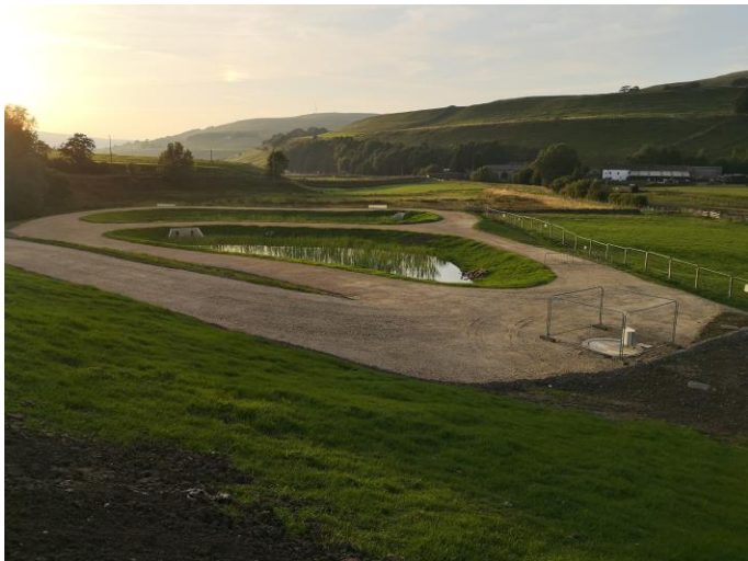
Reed beds at the Nent Hags mine water treatment scheme
