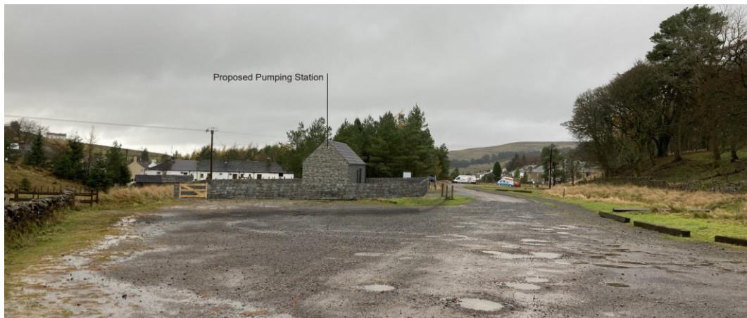
Visualisation of pumping station (option 5 is our preferred location) at the Nenthead car park
