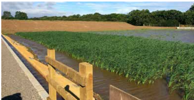
The wetland at Saltburn mine water treatment scheme
