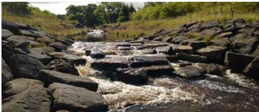
Example of existing sediment trap near Nenthead
