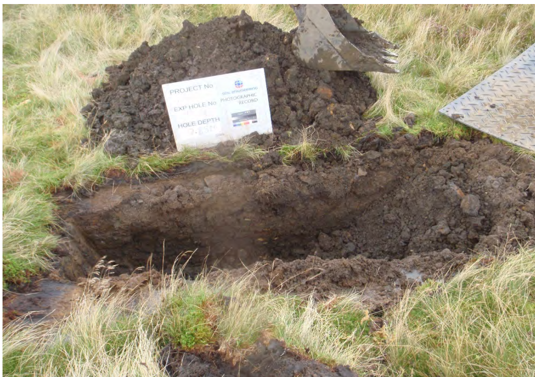
Photograph of Side C - 0.85m
