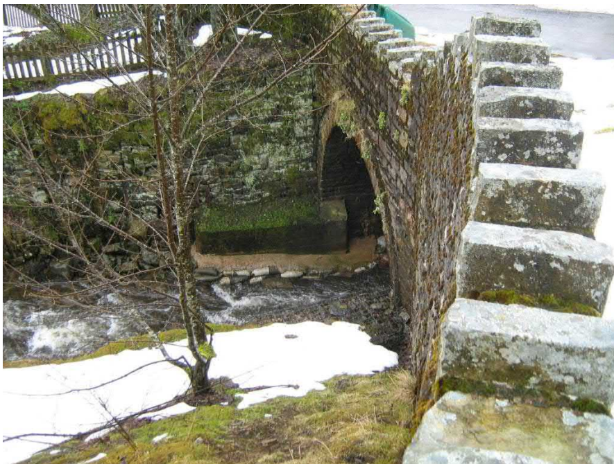
Photograph 18. Culvert of the River Nent.
