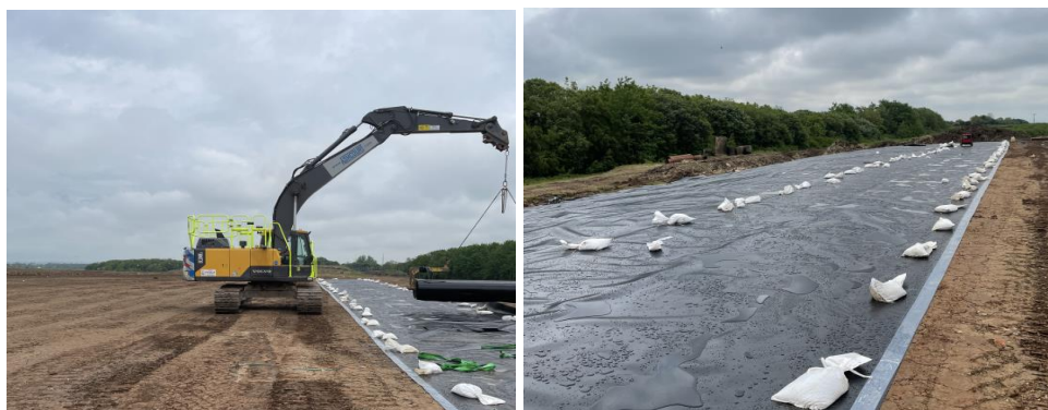
Images 2 & 3: Capping works in progress
