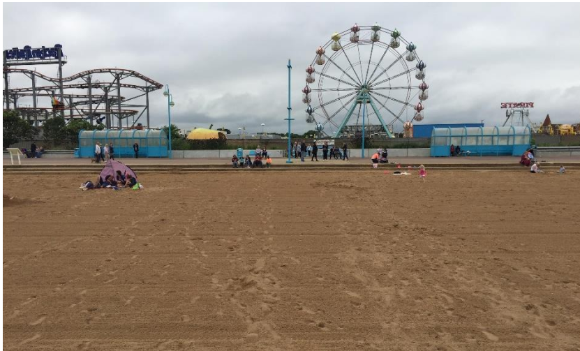
Plate 2.2: Skegness – North Bracing beach, promenade and flood wall (Zone B)
