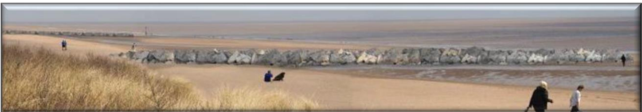
Visualisation of how a rock groyne may look on the licolnshire beaches
