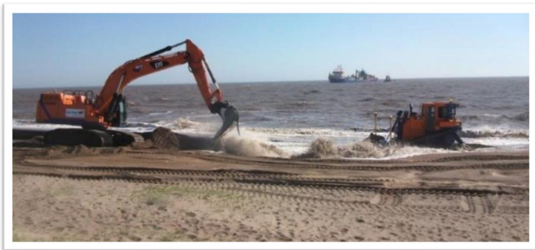
Beach nourishment operations – May 2016
