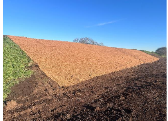
Winter Recovery repair works carried out at South Delph (Branston Fen)
