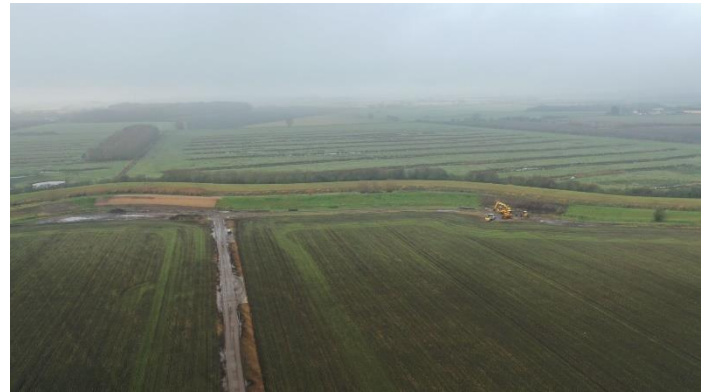
Photograph 2: Drone Image of Barlings Repairs 2020
