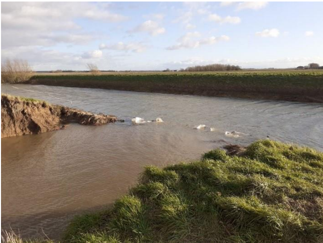
Photograph 1: Timberland Delph breach November 2019
