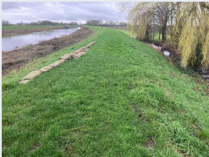
Embankment in the Lower Witham Fens (Kyme Eau).
