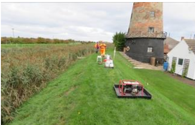
Figure 3: Slipped embankment upstream of railway bridge.
